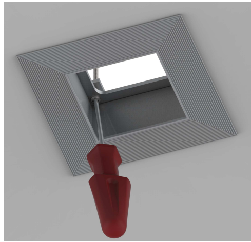
Step (8) Locking frame to drywall by tightening the support bracket screws
